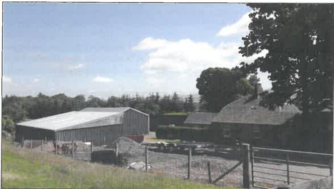
Fig 2: Sheds at Spylaw Steading
