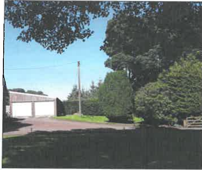
Fig 3: "Shed 3" (Garage) at Spylaw
